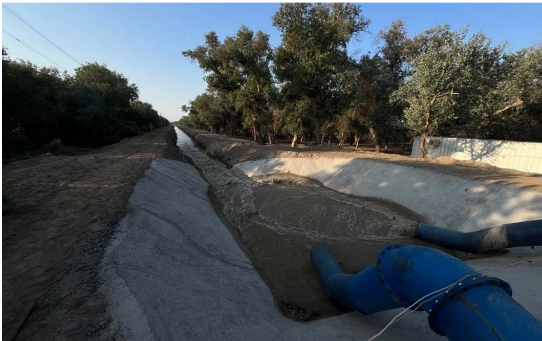
New canal and pumps to replenish the reserve's ecosystems
